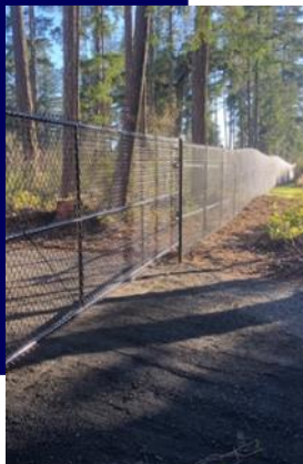
Chain link fencing around the remainder of our property
