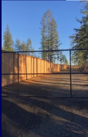
Cedar fence along the north property line was installed November 2020
